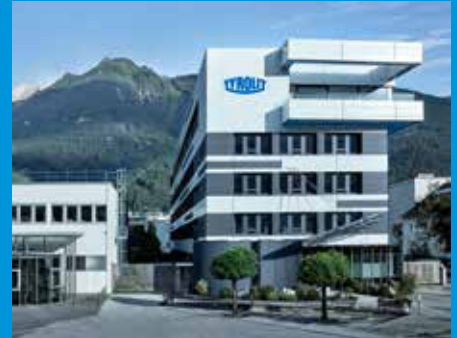
Tyrolit headquarters in Schwaz (Austria)
